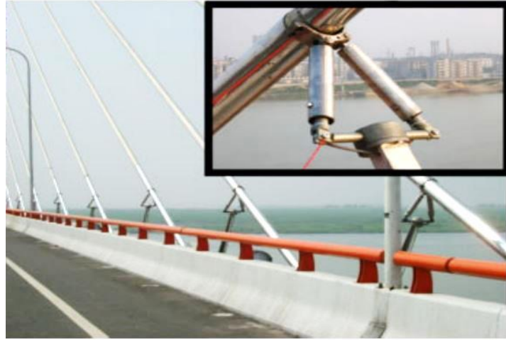
Figure 2.2 MR damper applied in structural damping (Wang et al. (2018))
