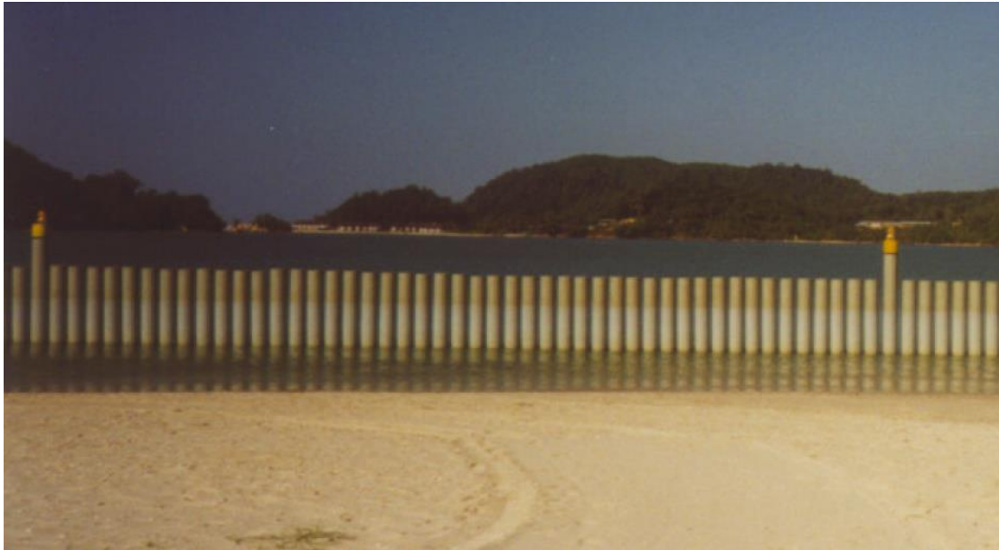
Fig. 1.2 Row of pile breakwater at Langkawi, Malaysia (Reedijk and Muttray 2009)
