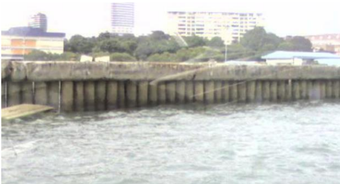
Fig. 1.3 Row of pile breakwater at Pasir Panjang, Singapore (Liu et al. 2011)
