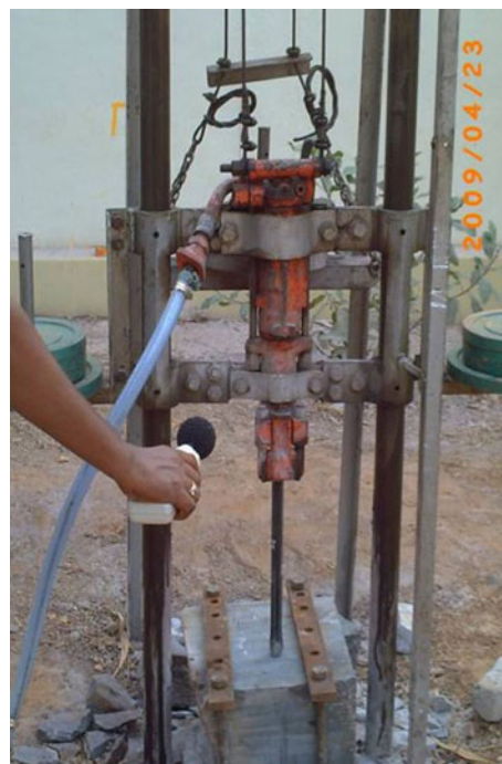
Fig. 1 Jackhammer drill setup for drilling vertical holes in rock samples
