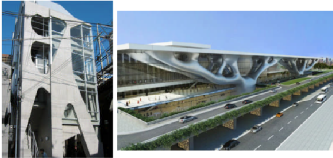
Figure 1.3: a) An office building in Japan with topology optimized Walls b) A topology optimized support structure(Source:Wikipedia)
