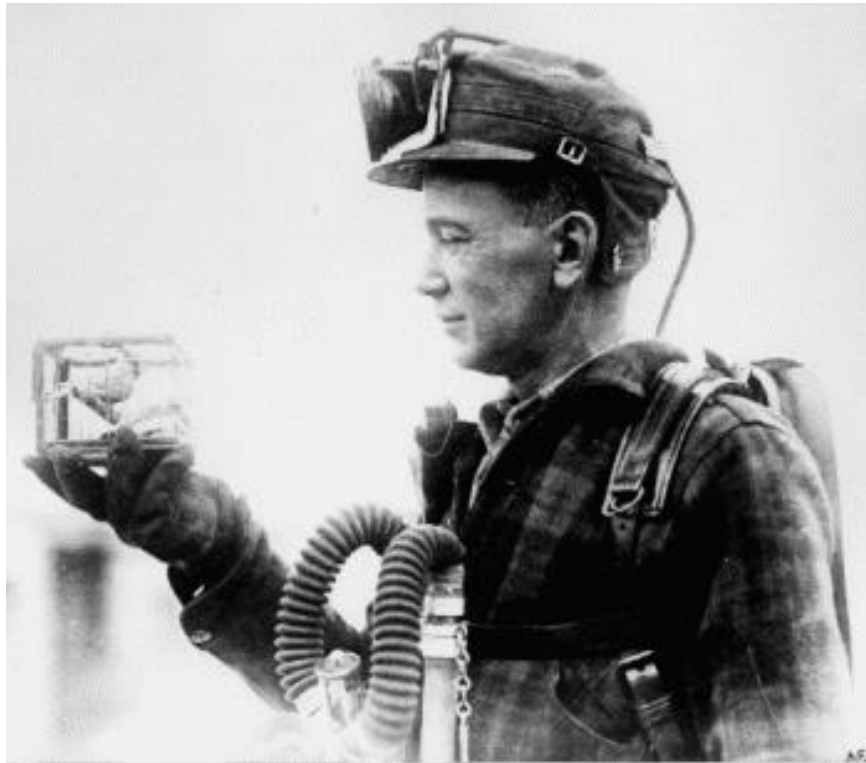
Fig. 2.2 Canaries served as an early warning system for miners in underground mines, (Kaur (2012))
