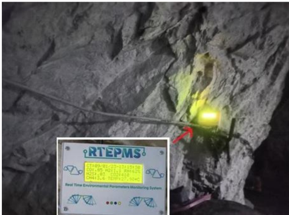
Fig. 5.27 RTEPMS with LoRa receiver deployment at tunnel 26 of the underground mine 'B'
