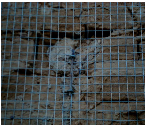
Fig.4 Steel wire mesh and tie against the adobe walls (Petrozzi, G R et al, 2014)
