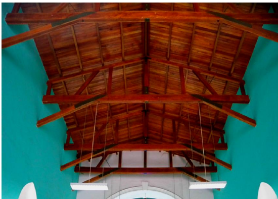
Fig.3 Reconstructed trusses (Petrozzi G R et al, 2014)
