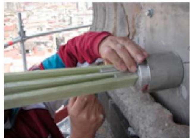
Fig.6 Installation of GFRP ties (Ceroni F et al, 2009)
