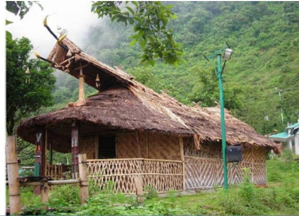
Fig 4(b).NAGA HOUSE WITH DOUBLE PITCHED ROOF
