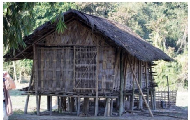
Fig 3. TYPICAL STILTED HOUSE
