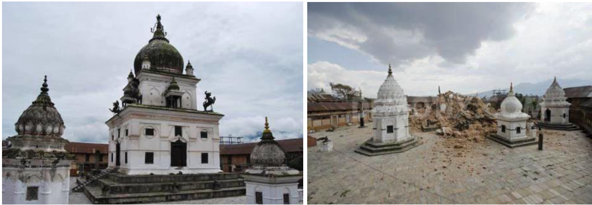
Fig.5 Kal Mochan Ghat: before and after (ICIMOD)
