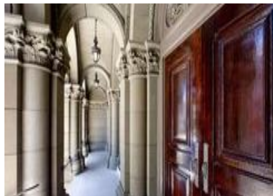
Fig.12 Restored wooden doors- (elsarch.com, 2012)
