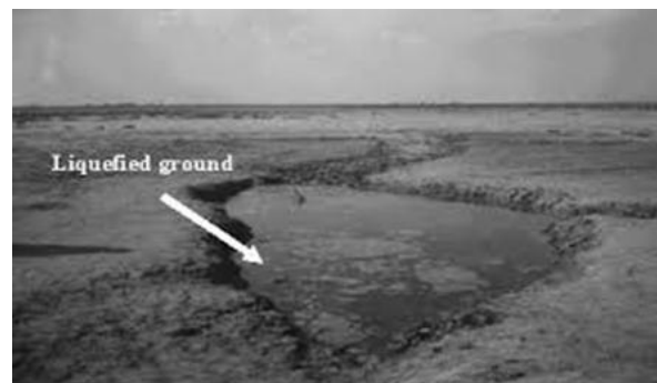
Figure 5. Liquefied Ground in Bhuj, January 2001 (Photo: Dr. T.G.Sitharam, IISc Bangalore)
