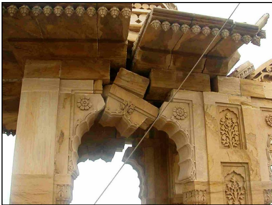
Fig.8 Destruction of Arches (Shethi, A. et al 2004)
