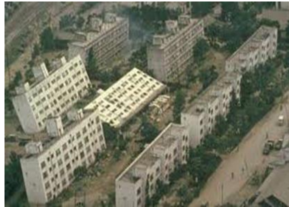
Figure 4. settlement during Niigata earthquake 1964, Japan
