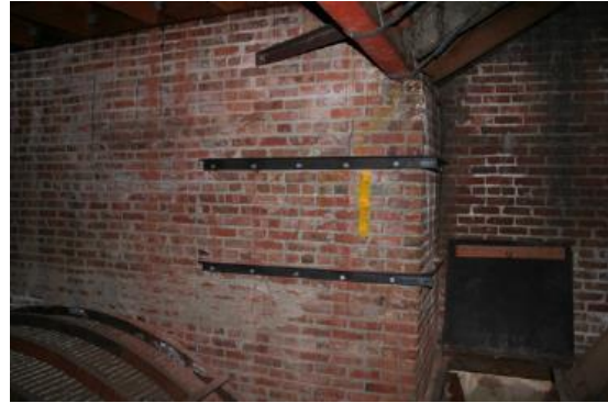
Fig.10 Steel angles to suture the walls (Paret T F et al, 2008)
