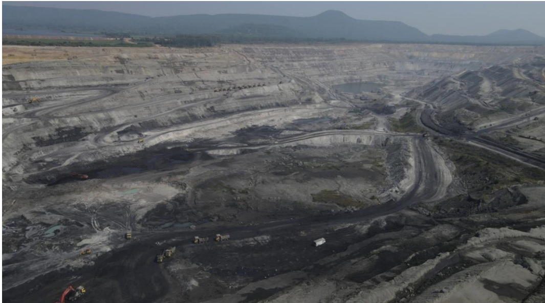
Figure 3.22 A view of KHG OC Coal Mine
