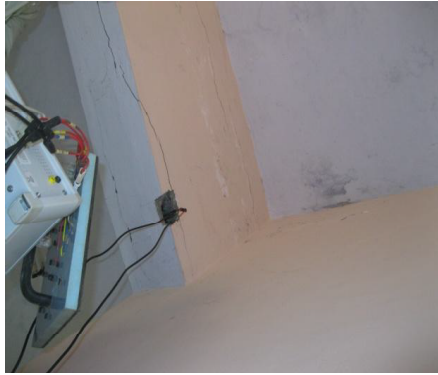
Fig.6.2: View of working electrode connection to rebar
