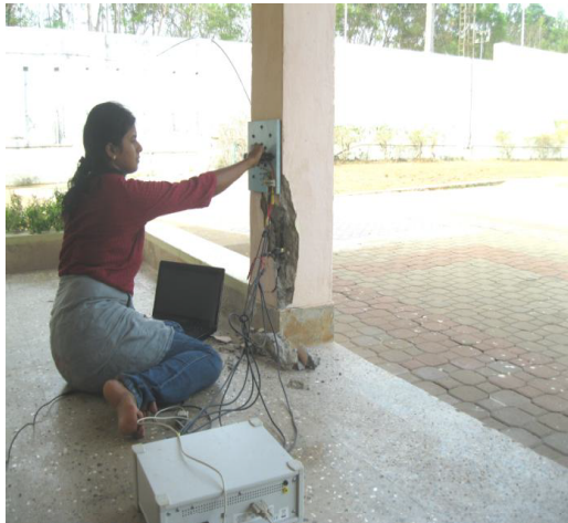
Fig.6.6: Monitoring of RC column
