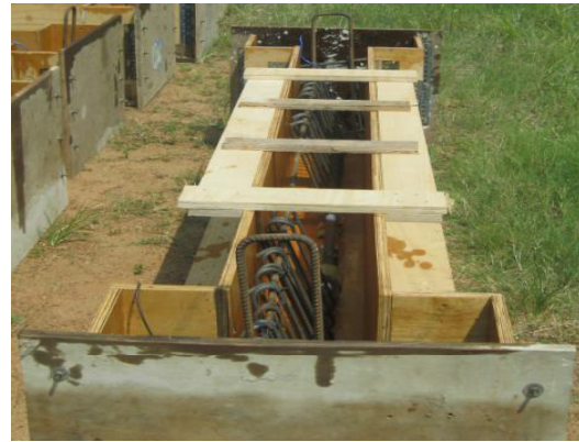
Fig. 3.13: Form work with reinforcement cage
