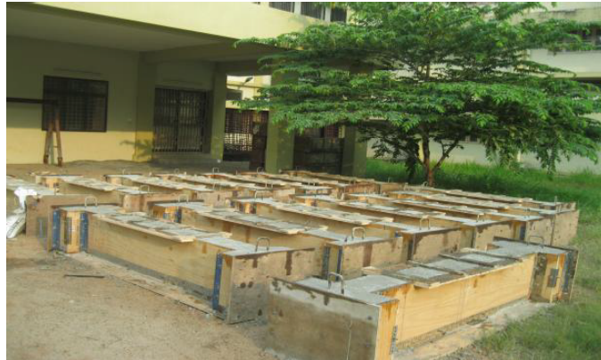
Fig.3.17: Concrete finishing work in NBS beam specimen moulds
