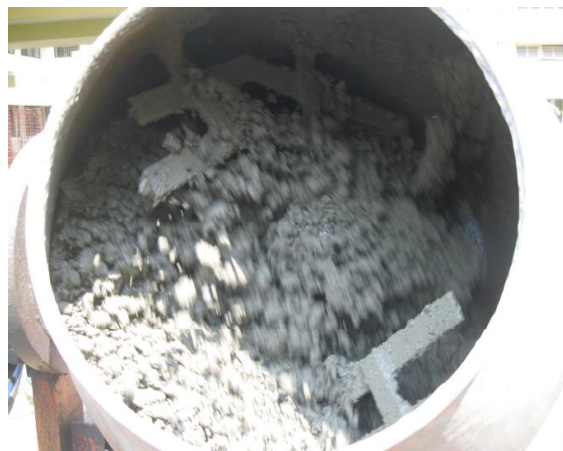
Fig.3.14: Mixing of concrete
