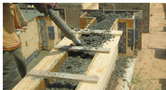
Fig.3.16: Compaction with needle vibrator
